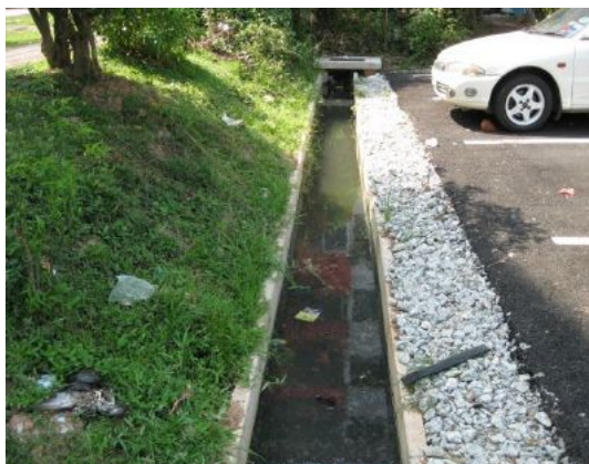
Gambar 2.5 Tiada Kerb Dibina
